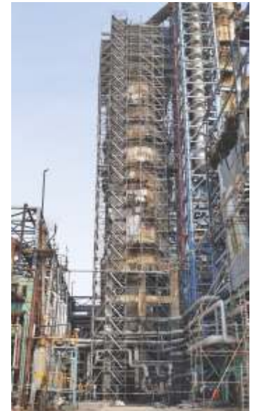
Layher Allround Application in Column Maintenance of Column in Refinery
